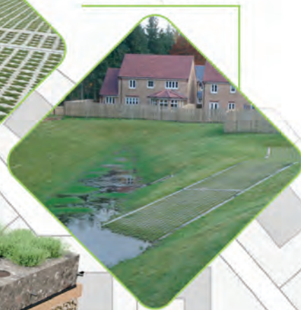
Grasscrete - water attenuation including SUDS
