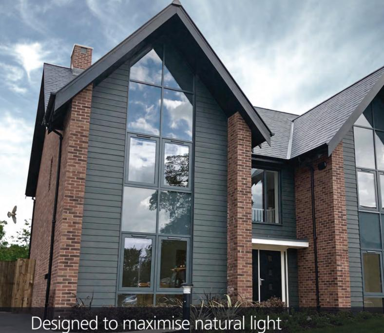
Commonly thought of as a commercial product, curtain walling is becoming increasingly specified for homes to create a light and airy living space. The architect specified the Kestrel Aluminium100mm box and plate curtain walling system incorporating Kestrel 60mm windows to maximise natural light and give a dramatic frontage to this prestigious development on the Coton House Estate, near Rugby.
