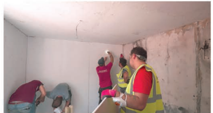
4: Removing burnt plasterboard, redecorating, fitting new electric sockets and new lights to existing cables.
