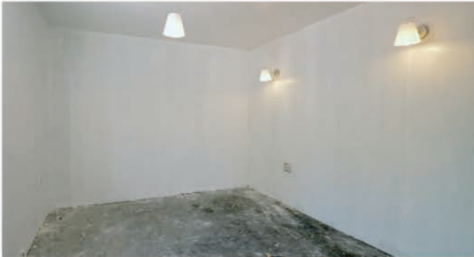
5: One of the burnt rooms rapidly and fully restored and ready for occupancy. Removal and replacement of burnt plasterboard and replacement of electric fittings took about 2 hours and 40 minutes.
