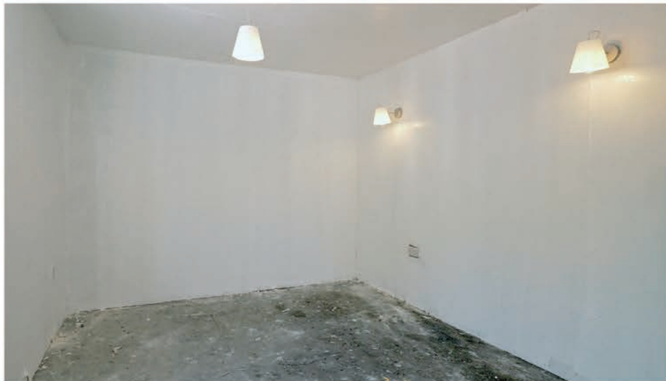
5: One of the burnt rooms rapidly and fully restored and ready for occupancy. Removal and replacement of burnt plasterboard and replacement of electric fittings took about 2 hours and 40 minutes.
