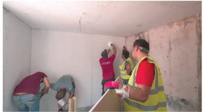
4: Removing burnt plasterboard, redecorating, fitting new electric sockets and new lights to existing cables.
