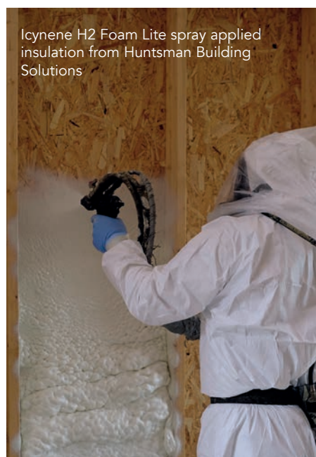
Spray applied insulation effectively seals the complex voids in a building structure.
