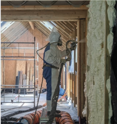
Huntsman H2 Foam Lite was sprayed to a depth of 230mm in the timber frame external wall and roof structure and 300mm at the roof/wall perimeter area.
