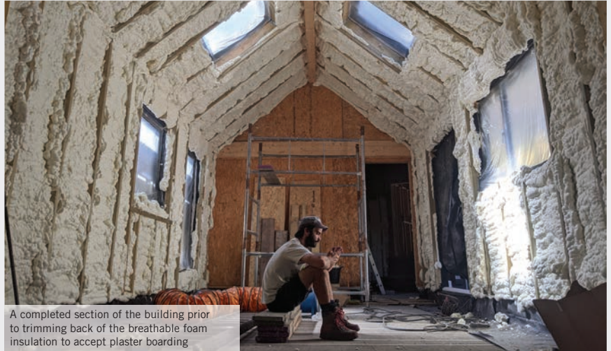
Huntsman H2 Foam Lite was sprayed to a depth of 230mm in the timber frame external wall and roof structure and 300mm at the roof/wall perimeter area.
