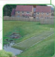
Grasscrete - water attenuation including SUDS
