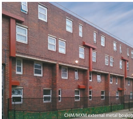
CHM/MXM external metal boxing
