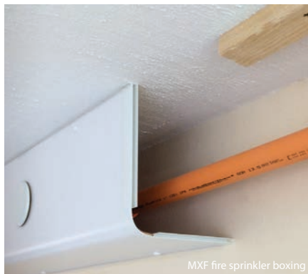
MXF fire sprinkler boxing
