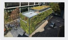
Biotecture's patented hydroponic BioPanel<sup>TM</sup> system is the most flexible, resilient, and low water use of any fully comprehensive living wall system anywhere in the world. A comprehensive independent engineering assessment with regards to reaction to fire confirms a system rating of B-s2,d0 which means the BioPanel<sup>TM</sup> living wall system can be retrofitted as part of a façade refurbishment and incorporated within new buildings as the integral rainscreen cladding element.
