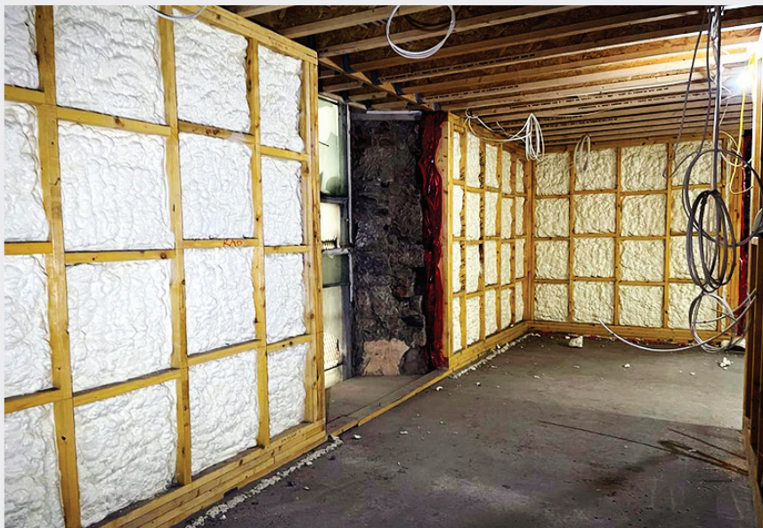
Insulation was applied to the inside of all external walls as well as the roof structure
