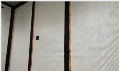
Installation of Delta MS 500 Fire Retardant, Type C waterproofing membrane system
