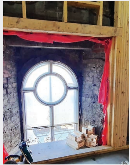
External walls were lined with timber studwork to accept insulation
