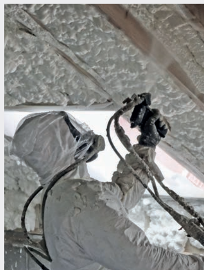
H2Foam Lite, a breathable spray foam insulation system from Huntsman Building Solutions
