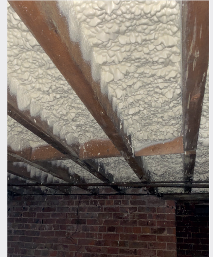
"The effect of using spray foam insulation in the cellar ceiling and roof space has been remarkable" Cellar under-floor area shown
