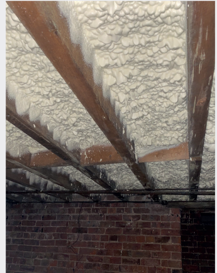
"The effect of using spray foam insulation in the cellar ceiling and roof space has been remarkable" Cellar under-floor area shown
