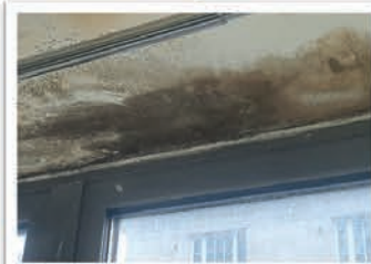
Water Ingress & Mould
