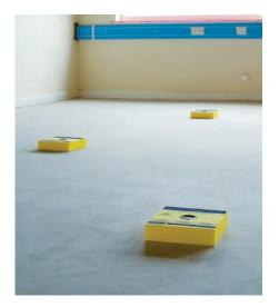
Digital hygrometers are affixed to the subfloor at regular intervals to accurately measure subfloor relative humidity (RH) levels
