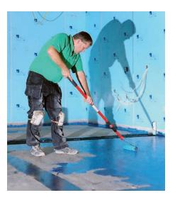
A fast-track liquid waterproof surface membrane can be used to create a barrier against residual construction moisture where relative humidity levels are up to 95%
