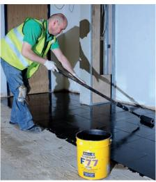
Application of a liquid waterproof surface membrane with a roller
