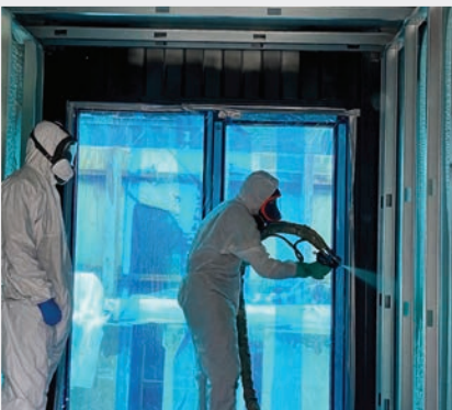
Heatlok spray foam insulation completely encapsulates the studwork and adheres to the contours of the metal container shell, eliminating the risk of condensation
