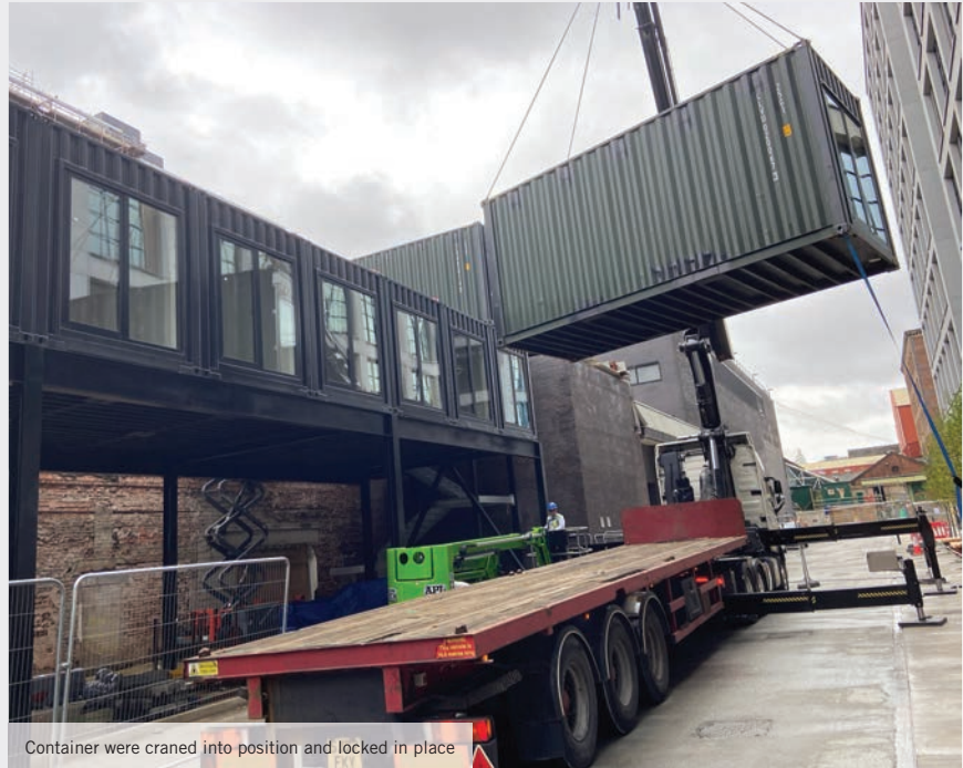
Containers were craned into position and locked in place
