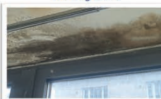
Water Ingress & Mould
