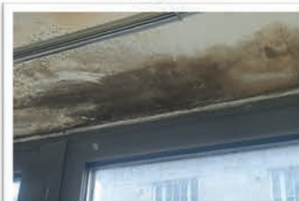
Water Ingress & Mould
