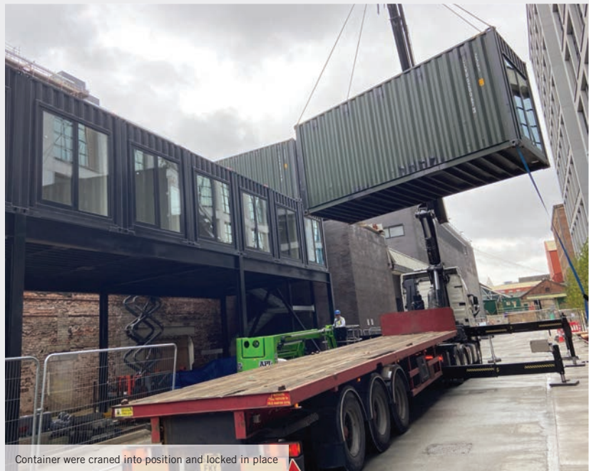
Containers were craned into position and locked in place
