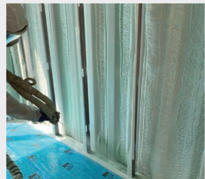
Heatlok expands 100-fold on application, completely filling difficult to reach construction voids and creating a continuous, uninterrupted thermal barrier
