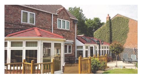
formed from lightweight aluminium and pre-insulated to ensure good thermal performance. Warm roofs are designed specifically for conservatories, and are usually preassembled in dedicated facilities bespoke to a conservatory's specifications.
