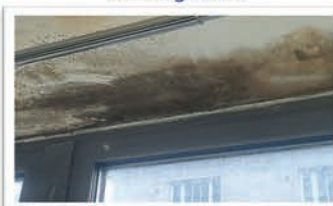
Water Ingress & Mould
