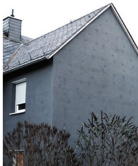
Anchor marks visible on the rendered facade of a property treated with an external wall insulation system
