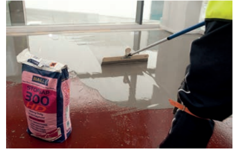
A smoothing compound is recommended to create a perfectly smooth base
