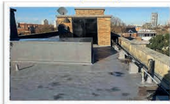
Flat & Commercial Roof Leaks
