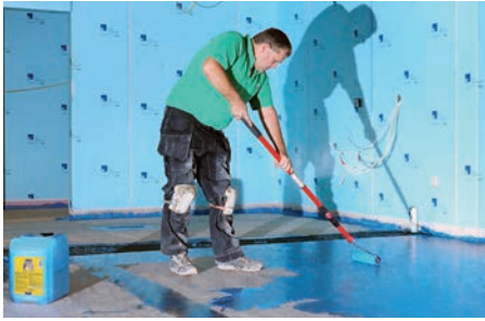
F. Ball's 'Fast-Track' Stopgap F78 waterproof surface membrane
