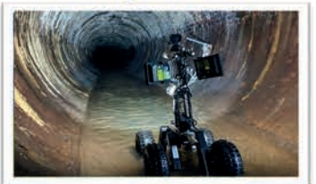
CCTV & Drone Surveys
