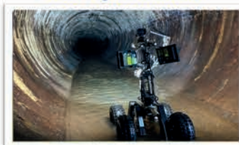
CCTV & Drone Surveys
