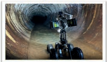
CCTV & Drone Surveys
