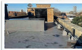
Flat & Commercial Roof Leaks
