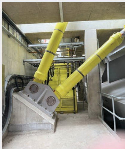
LIEBIG Ultraplus anchors securely angled to support the hydraulic mechanisms of the bridge decks as well as the tail locks that hold the Herring Bridge in its raised and open position.
