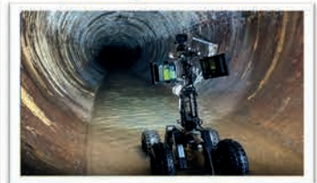
CCTV & Drone Surveys
