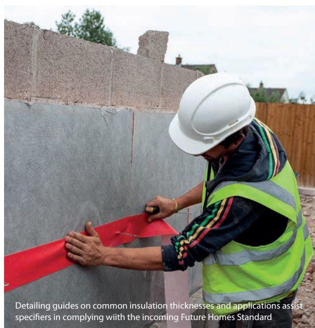
Thermal conductivities down to 0.019 W/mK are achievable with Kooltherm insulation
