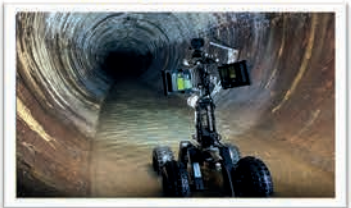
CCTV & Drone Surveys
