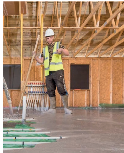
The common method for including UFH in a new build home is to include pipework in the floor screed
