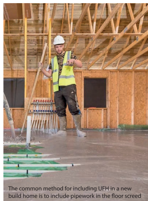
An underfloor heating pipework design
