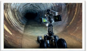
CCTV & Drone Surveys
