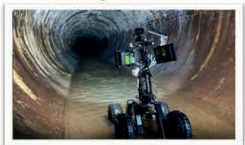
CCTV & Drone Surveys
