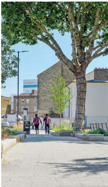
A new pocket park includes 'sponge city' principles with retrofitted permeable paving linked to green infrastructure © Robert Bray Associates
