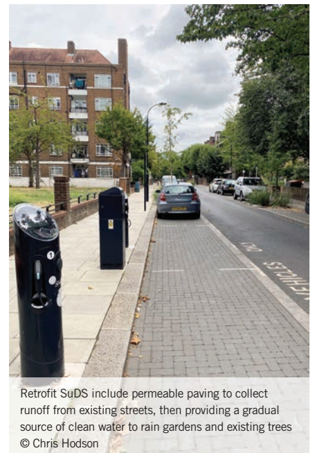
Concrete block permeable paving overlay on an existing road base conveys water to tree-planted basins © Robert Bray Associates
