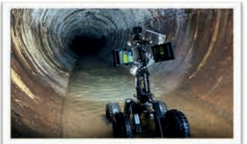
CCTV & Drone Surveys
