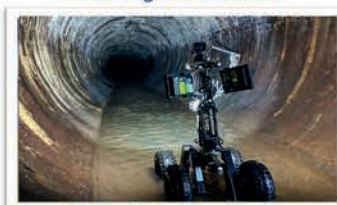
CCTV & Drone Surveys
