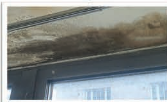
Water Ingress & Mould
