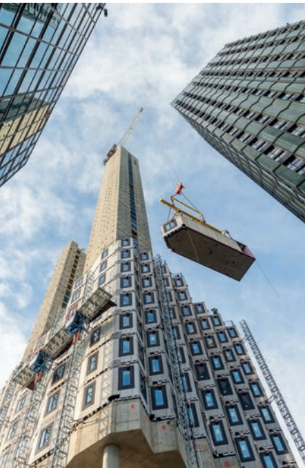
The largest module, fitted with bathrooms and kitchens, weighed up to around 30 tonnes
