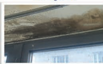
Water Ingress & Mould
