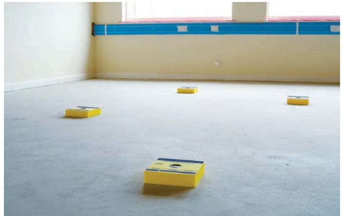
Digital hygrometers affixed to the subfloor at regular intervals to accurately measure subfloor relative humidity (RH) levels
