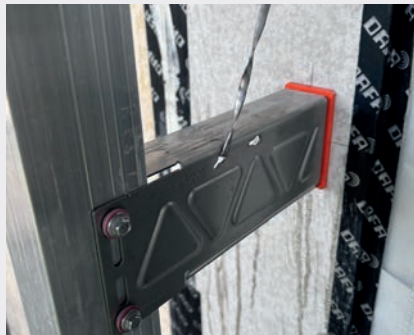
The CROSSFIX Konsole's stainless steel composition and thermal stop contributed to achieving the façade's 0.13 W/m 2 K U-value.
