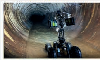
CCTV & Drone Surveys
