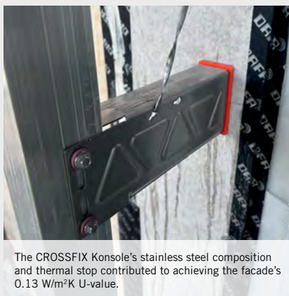
CROSSFIX enabled the use of two different types of cladding to be used, including secret-fix panels for the ground and first floors.
