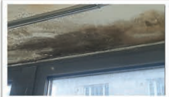
Water Ingress & Mould
