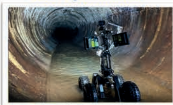
CCTV & Drone Surveys
